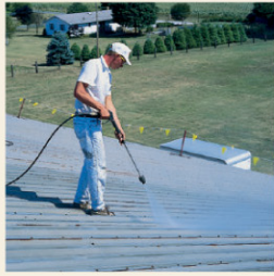
1. Power wash and clean with Rust Off®.
